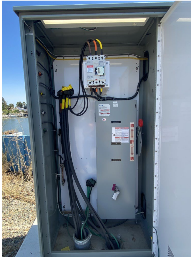
Figure 4. MTS located in Cabinet 1
