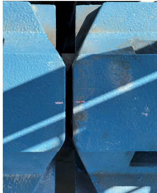
Figure 3. Markings on Gate Leaves, Miter Point
