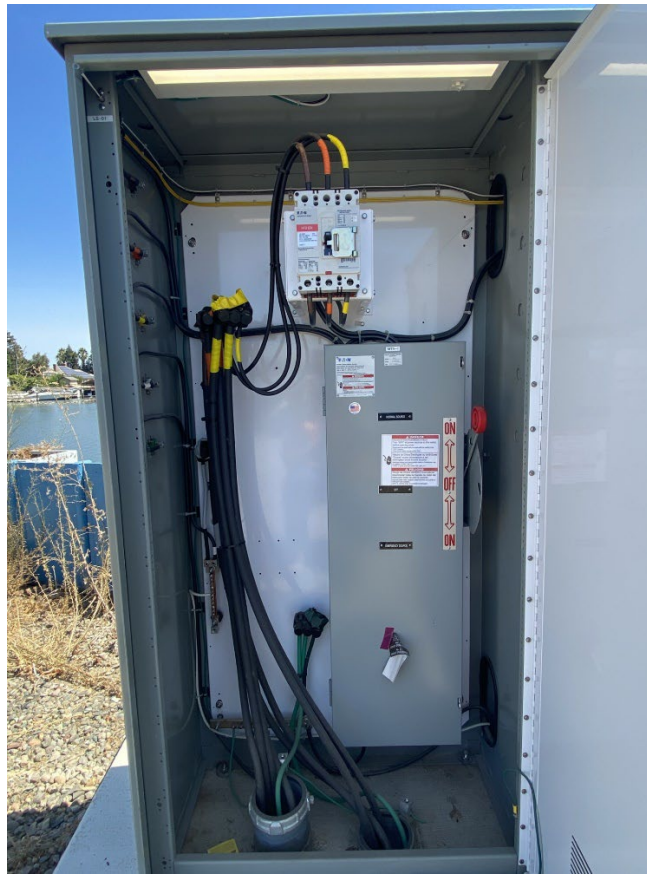
Figure 5. MTS located in Cabinet 1
