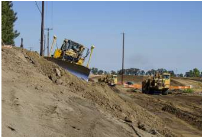
Bulldozer with GPS
