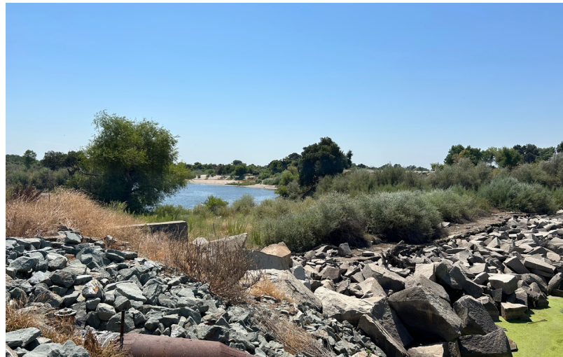
Existing Paradise Cut rock weir (July 2024)
