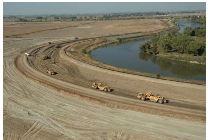
Construction of super levee - 2006
