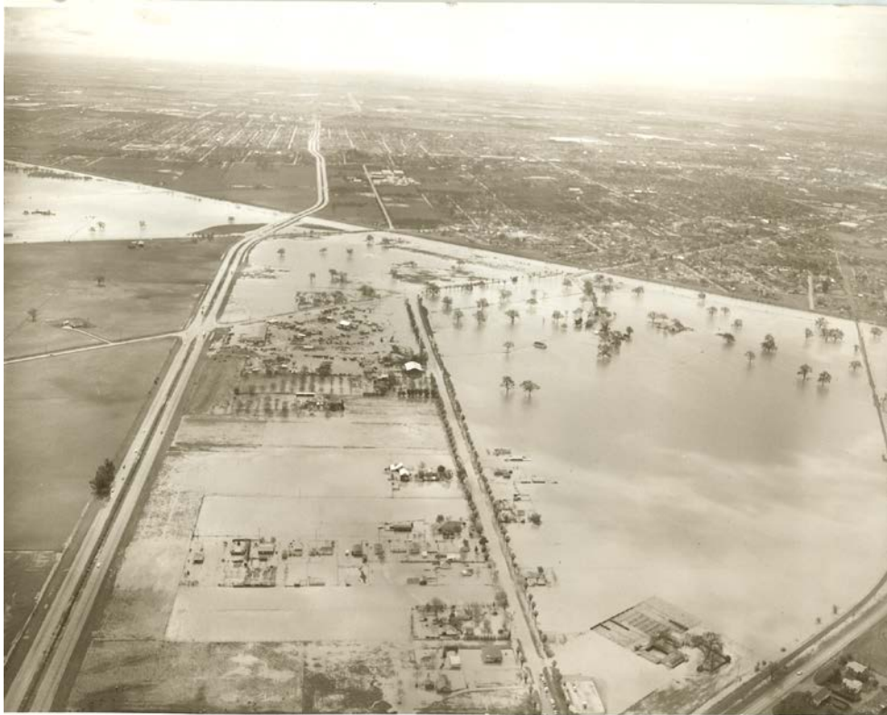
1958 Inundation from Diverting Canal (see Figure 7 for location)
