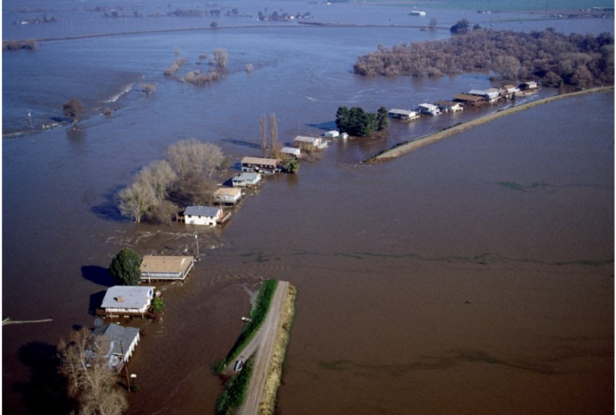
Image 7: Houses near a breach in RD 2075 levee in January 1997.
