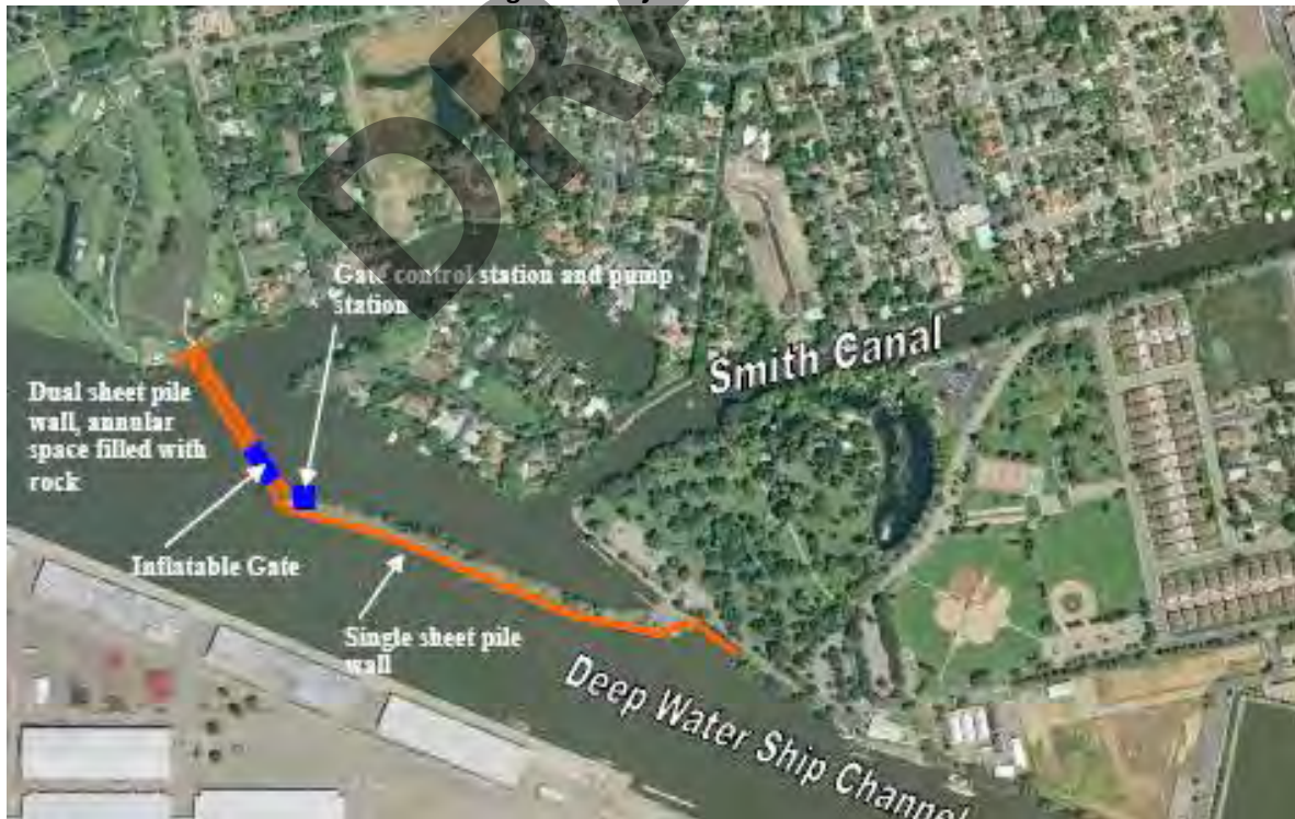
Figure 1: Project Aerial View
