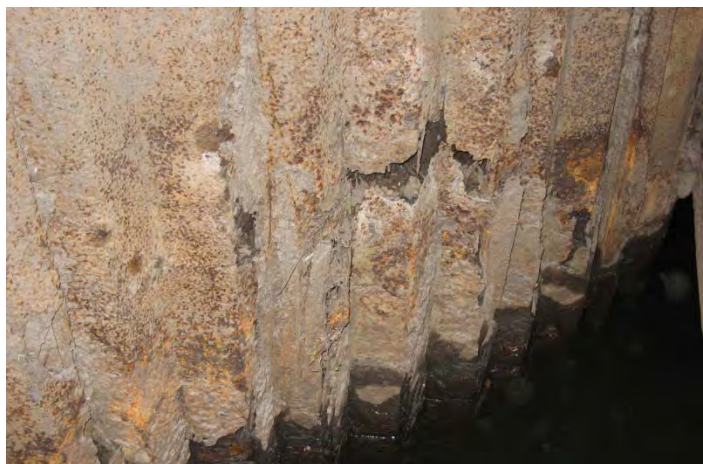
Figure 3. Photograph of Existing Sump Structure
